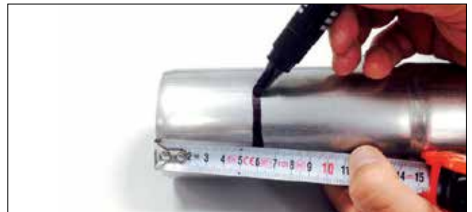
Figure 5 - Marking the insertion's depth
